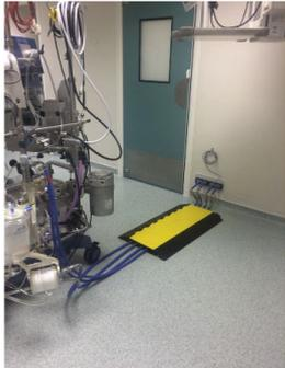
Figure 7. Position of the tubing through the wall into the operating theatre, using anti-slip matt housing and connection to the cardiopulmonary bypass equipment.
