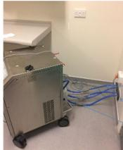
Figure 6. Positioning of the heater-cooler unit outside the operating theatre with tubing passing through modular plates in the wall.
