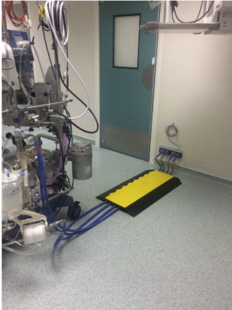
Figure 7. Position of the tubing through the wall into the operating theatre, using anti-slip matt housing and connection to the cardiopulmonary bypass equipment.
